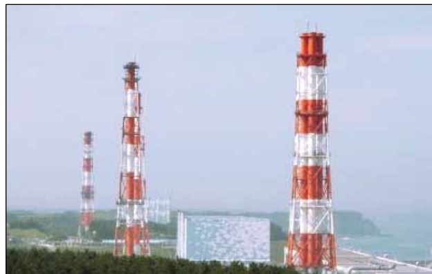
The Fukushima Daiichi Nuclear Power Plant in 2002
